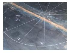
1. Draw the spiral staircase in real size on the floor to check the measurements and distances between steps.
