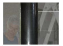
3. The top of each step is marked on the central tube of the staircase.
